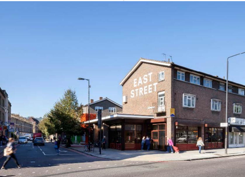
Navigational flank wall signage in Walworth, London
