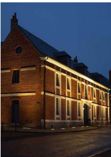
Lighting to enhance historic building features and detail
