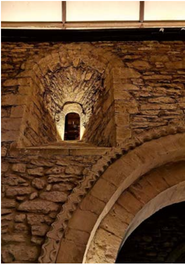
Lighting to highlight specific heritage features
