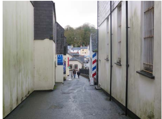
Flank walls within allyway leading to Dennison Road car park, currently covered in green algae
