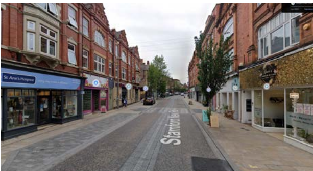
Stamford New Road, Altrincham: pedestrian priority street with narrow carriageway at level with pavement and street trees
